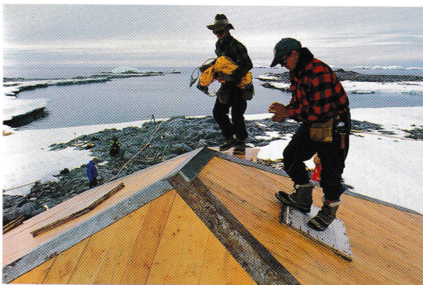
The new roof showing the huts proximity to Boat Harbour.
