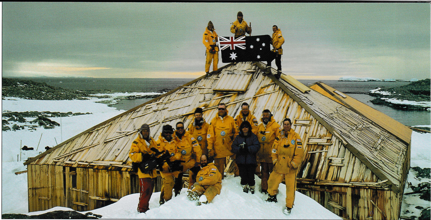
The AAP Mawson's Huts Foundation team pictured (left to right) on the roof of Mawson's Hut are carpenters David Gillott, Paul Delaney and Ted Bugg. On the ice in front of the hut are film cameraman Malcolm Ludgate, director Mike Piper, Joan Russell, Dr Rod Givney, Allen Rooke, David Killick, Alan Grant and Geoff Ashley. In front of them are Alasdair McGregor and Dr Estelle Lazer.
