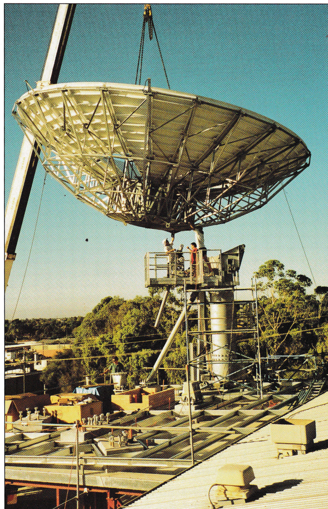
The PanAmSat contract involved the installation of two new 11-metre and one 4.5 metre antennae at Bayswater in Perth and an 11 metre, 6.8 metre and 4.5 metre antennae in Adelaide. Our picture shows the two large dishes being positioned at the AAPT earth station facility at Bayswater. Electronics systems within the facility provide for remote monitoring and control, telecommanding, ranging and telemetry reception.
