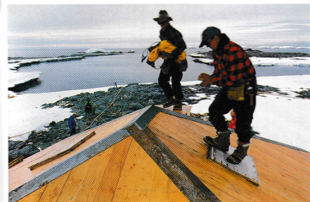
The new roof showing the huts proximity to Boat Harbour.
