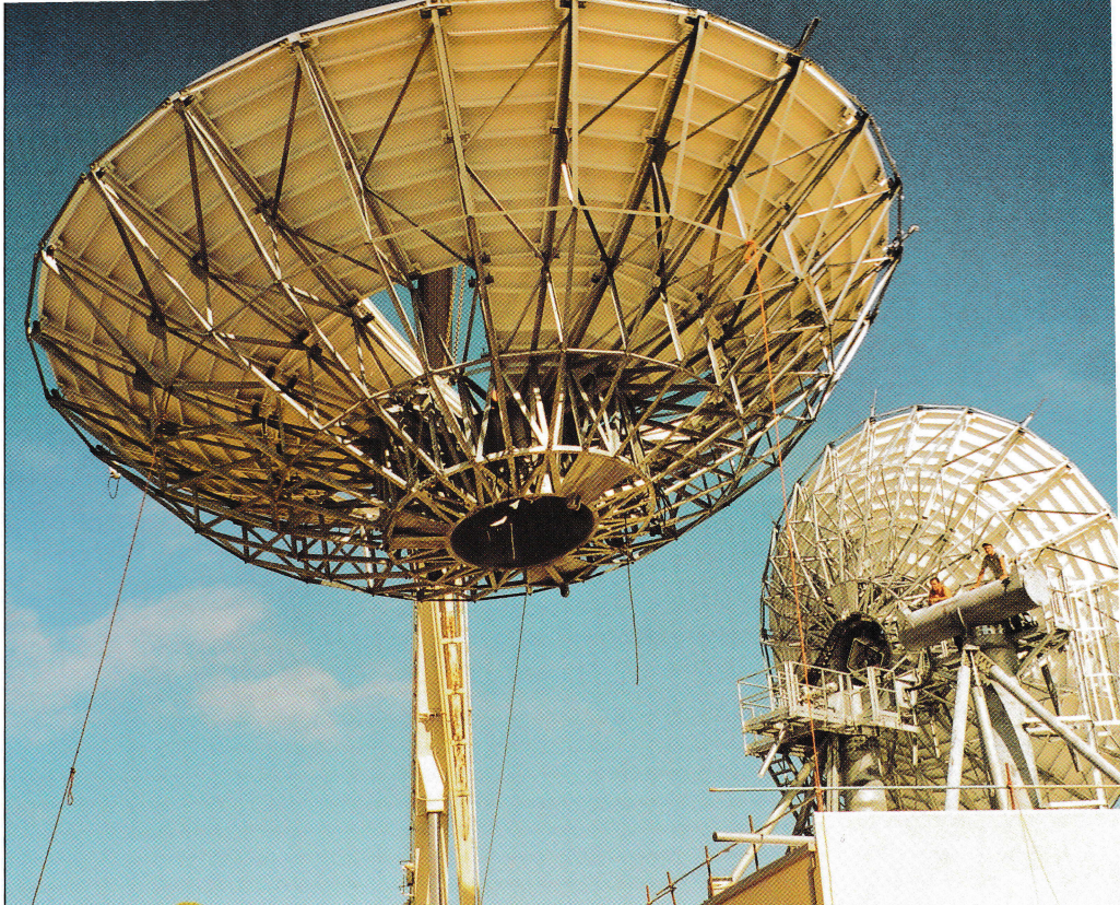
The PanAmSat contract involved the installation of two new 11-metre and one 4.5 metre antennae at Bayswater in Perth and an 11 metre, 6.8 metre and 4.5 metre antennae in Adelaide. Our picture shows the two large dishes being positioned at the AAPT earth station facility at Bayswater. Electronics systems within the facility provide for remote monitoring and control, telecommanding, ranging and telemetry reception.
