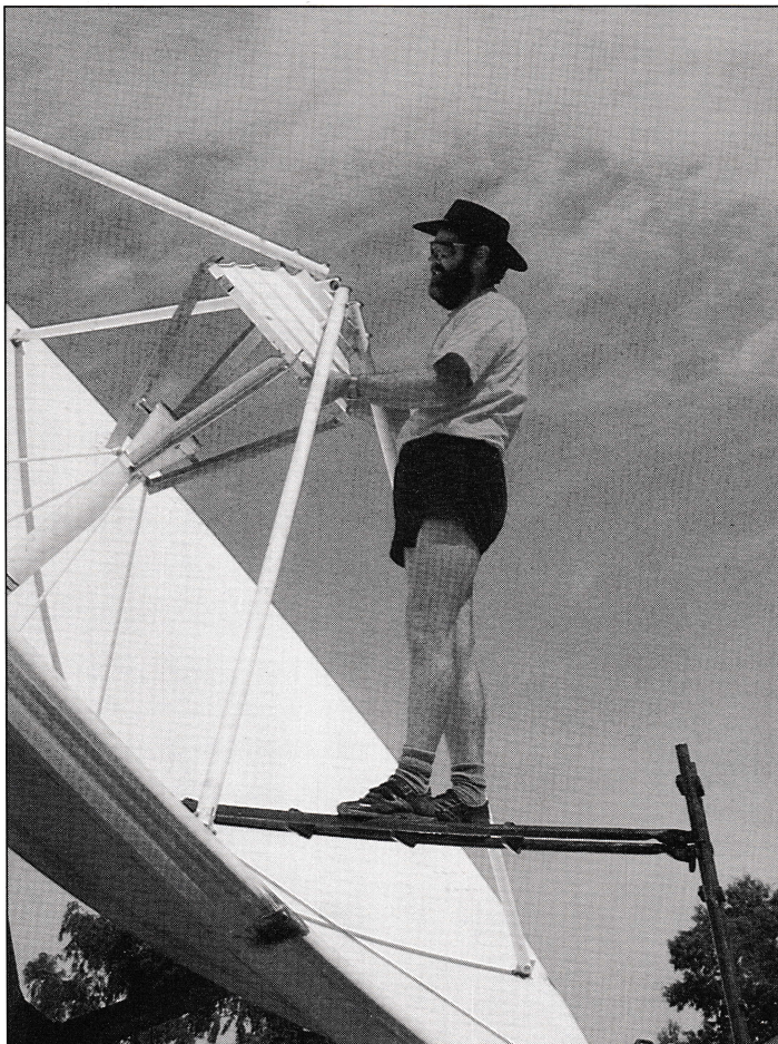
Garry Dawson hard at work installing part of the Tanami network.
